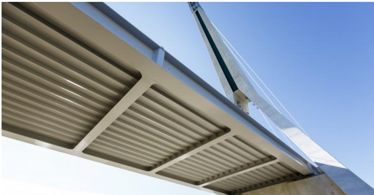
Figure 34. Steel bridge decking
