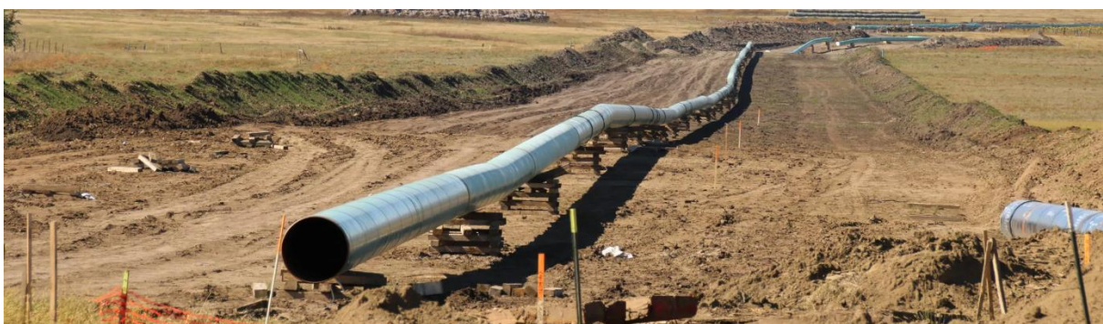
Figure 35. Conventional pipeline installation.
