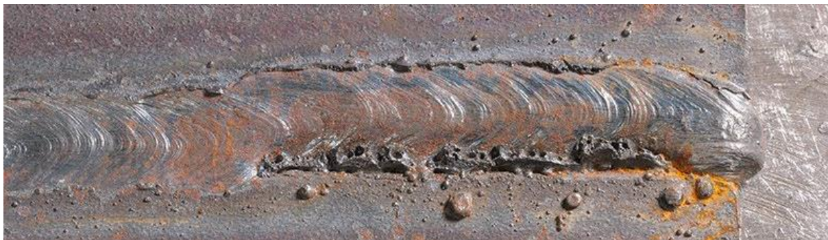
Figure 30. Surface of an arc weld showing spatter and unevenness.
